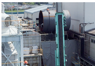
Unit 8 rotary kiln exchange
