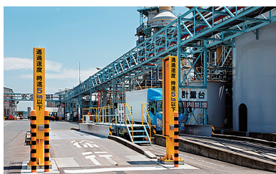
Measuring equipment. The yellow pillars next to the weighing equipment are radiation measuring instruments. They measure the radiation level of waste brought into the facility
