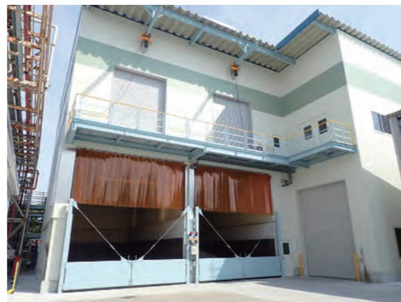
The expansion from one dehydrator to two, instead of the previous one, has contributed to stable operation. (Photo: Expanded dehydrator building)
