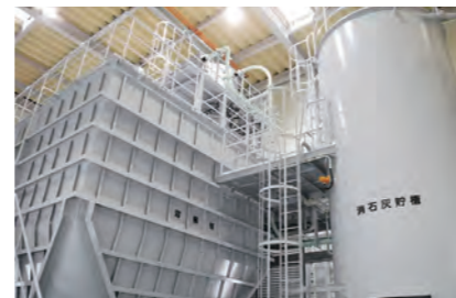
"Honestlimer", equipment that injects a solution of calcium hydroxide
